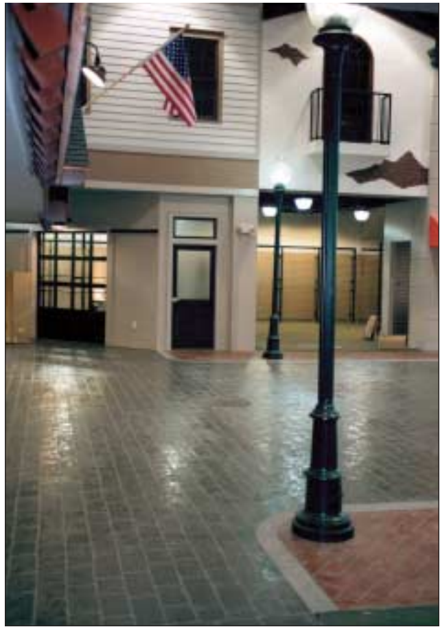
Tightening volatile organic compound (VOC) laws have made water-based sealers and coatings increasingly popular for protecting decorative concrete.
