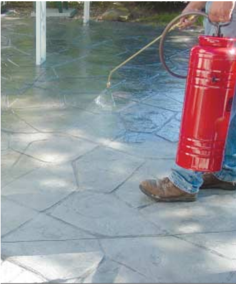
Treating decorative concrete with a sealer or coating can inhibit the penetration of water, chlorides, oils, and most other liquids, while enhancing the finish.
