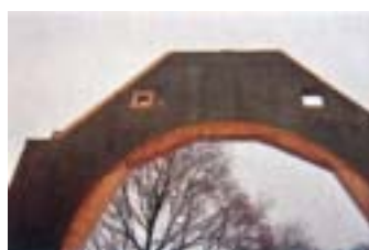
Fig. 1: Archway that was to become the new entryway to Greenfield Village (part of the Henry Ford in Dearborn, MI). Freeze-resistant concrete allowed placement in the middle of winter while maintaining a 7 in. (175 mm) slump
